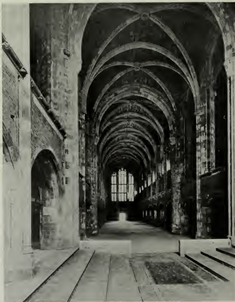
INTERIOR OF CHAPEL AT WEST POINT. Gothic vaulted ceiling of Guastavino construction. Cram, Goodhue & Ferguson, Architects.
